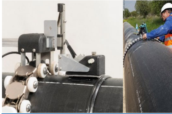
Polyethylene pipe weld inspection
