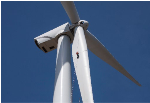
WTG Blade Root inspection
